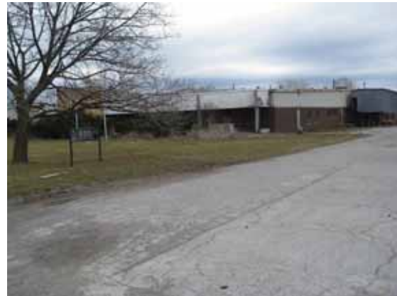
Plate 2: View southeast across entranceway and graded lawn toward industrial building. Area is all disturbed and has no potential.
